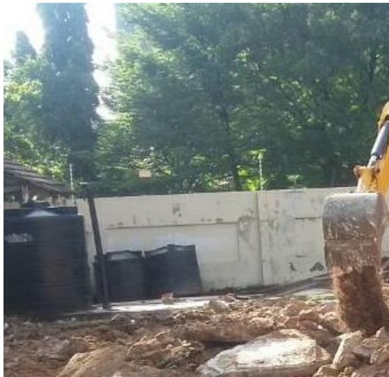
Figure 3 Site clearing after demolition
