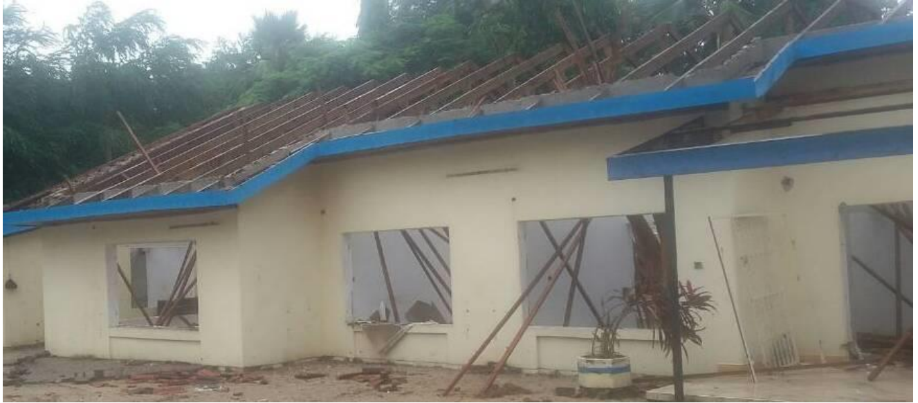
Figure 2 Demolition of TLS House on plot 391
